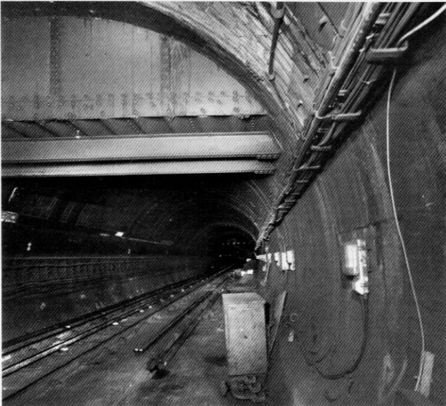
Site of the South Kentish Town northbound platform. Photo Nick Catford
